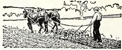
HARROW, McCORMICK-DEERING, SPRING TOOTH, WITH LEVERS
